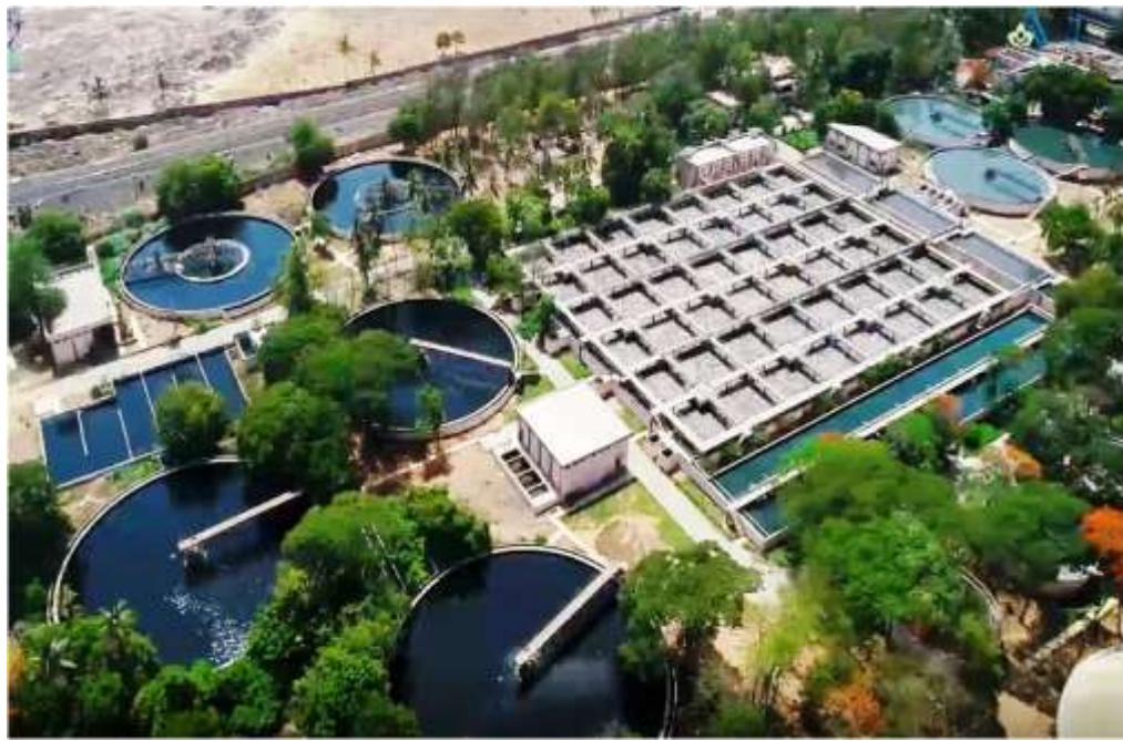
Anjana Sewage Treatment Plant
