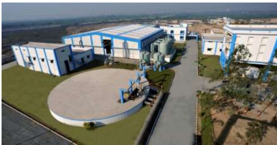
Bamroli Tertiary Treatment Plant
