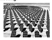
Since sunlight is not concentrated in one place, solar energy needs to be collected. Solar power plants can capture a lot of energy since their collection devices are laid out over large, flat, open, sunny areas.
